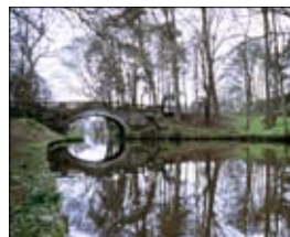
Canal bridge at Ellel Grange
